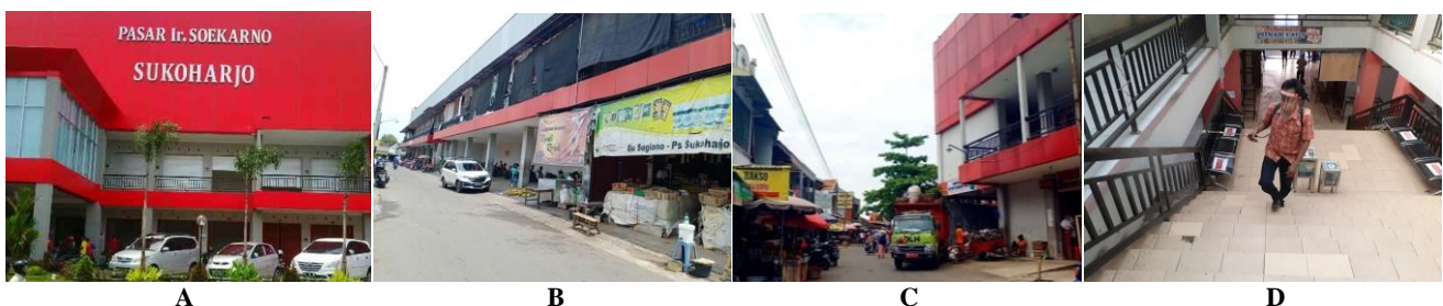
Figure 2. The Ir. Soekarno Market Building, Sukoharjo District, Central Java Province, Indonesia. A. Front view, B. Back view, C. Side view, D. Inside view
